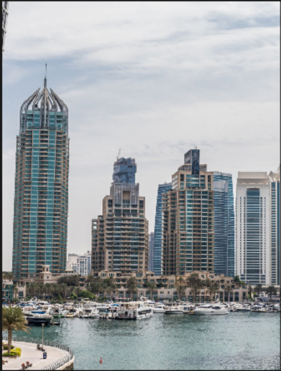
Civil & Structural Works
